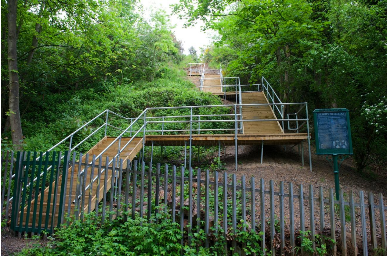
Steps erected on the east face
