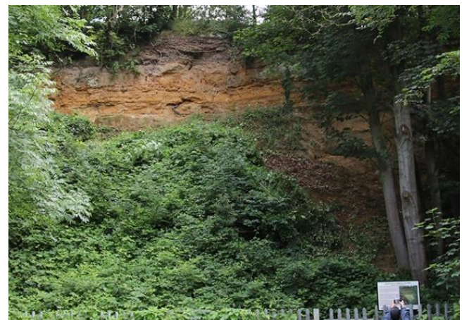
South face after clearing brambles but some left to keep face stable
