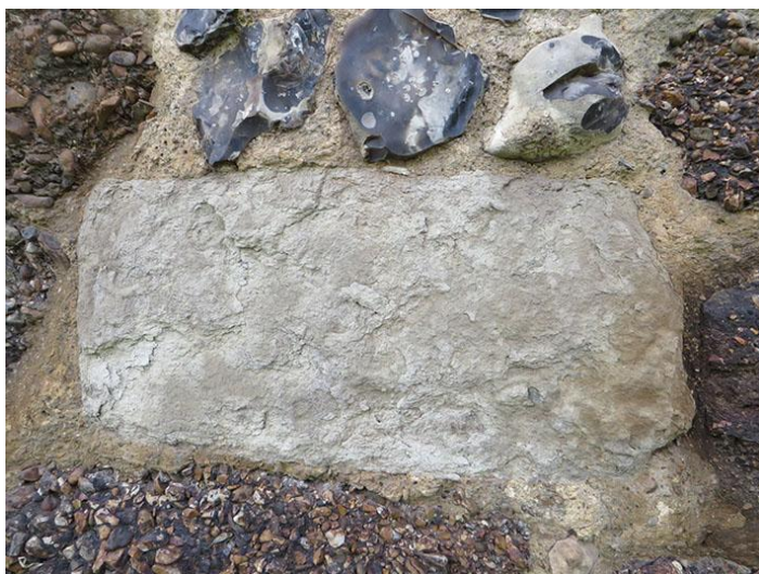
Reigate Stone and flint nodules used in the rubble masonry of the Harmondsworth Great Barn foundation walls.
