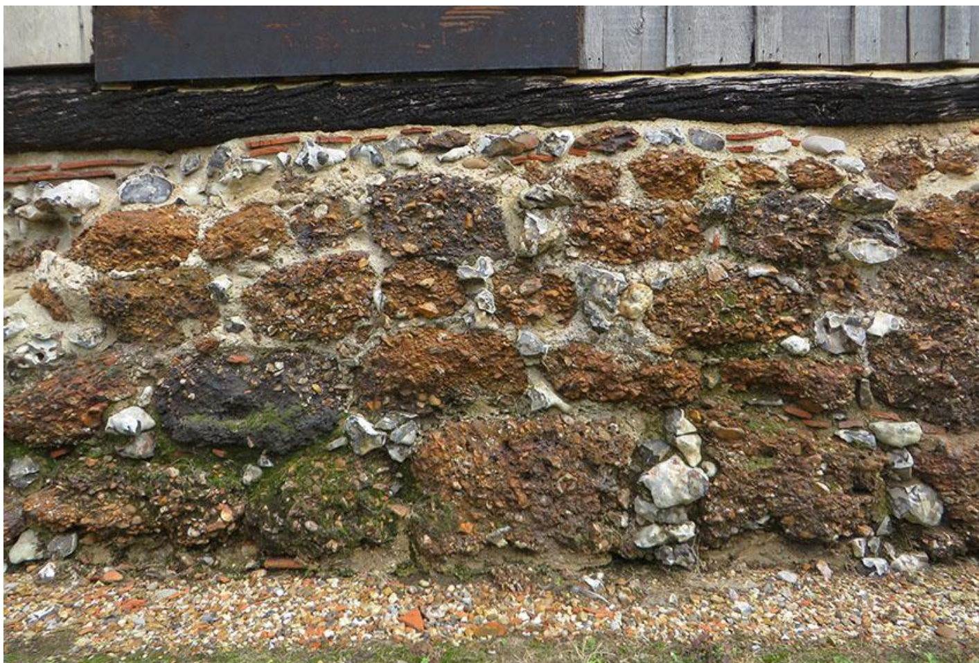
Foundation walls of Harmondsworth Great Barn.
