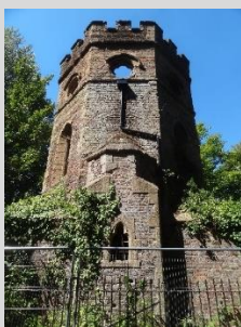
Gothic style tower used as boathouse on Potomac Lake, built on the foundations of a kiln, 11.8.2022.
