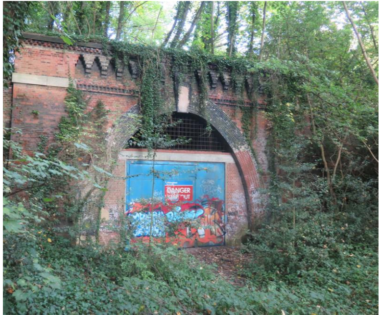
Southern portal to Crescent Wood Tunnel (TQ 3423 7201)
