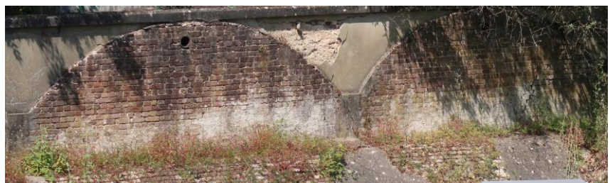
Arches, all that remain at site of Rock Hill reservoir
