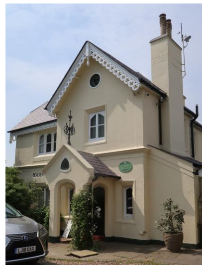
Tivoli Lodge, the entrance to Beulah Spa. Photo: L Baker
