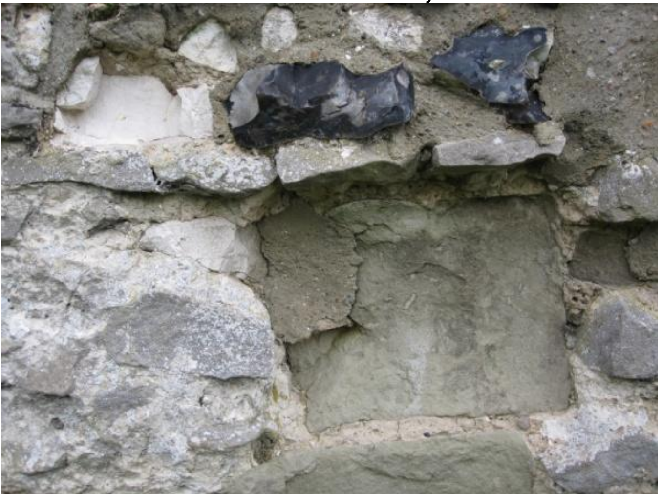
Close-up of wall Photos: D. Clements
