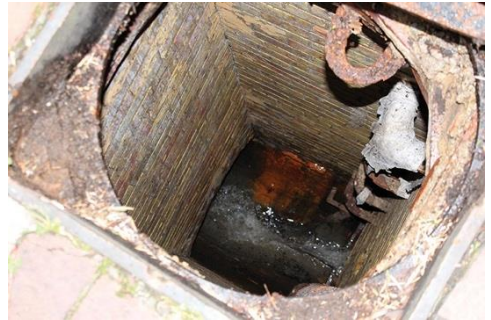
The Westbourne can be heard coming from the drain at this point even when it's covered. Photo Arup
