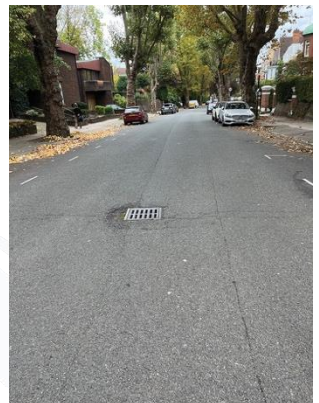
Drain in middle of Heath Drive. Redington Froggnal Association, 2025
