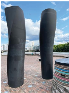
The new Chelsea Quay in 2025 with a view between the ventilation shafts to Chelsea Bridge and the refurbished Battersea Power Station beyond. Note the layered brickwork of the Florian Roithmayr design.
